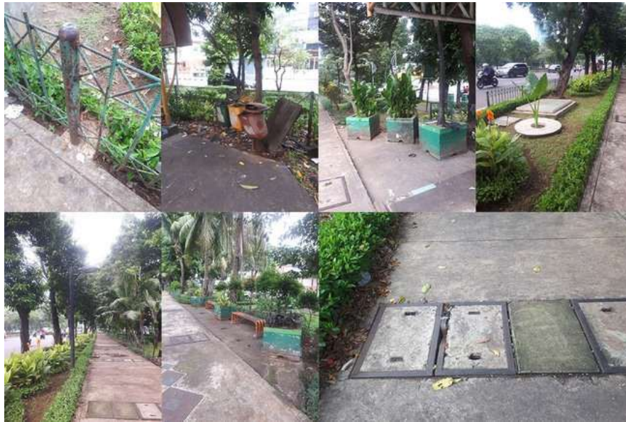
Figure 4. Existing condition of the study area.
