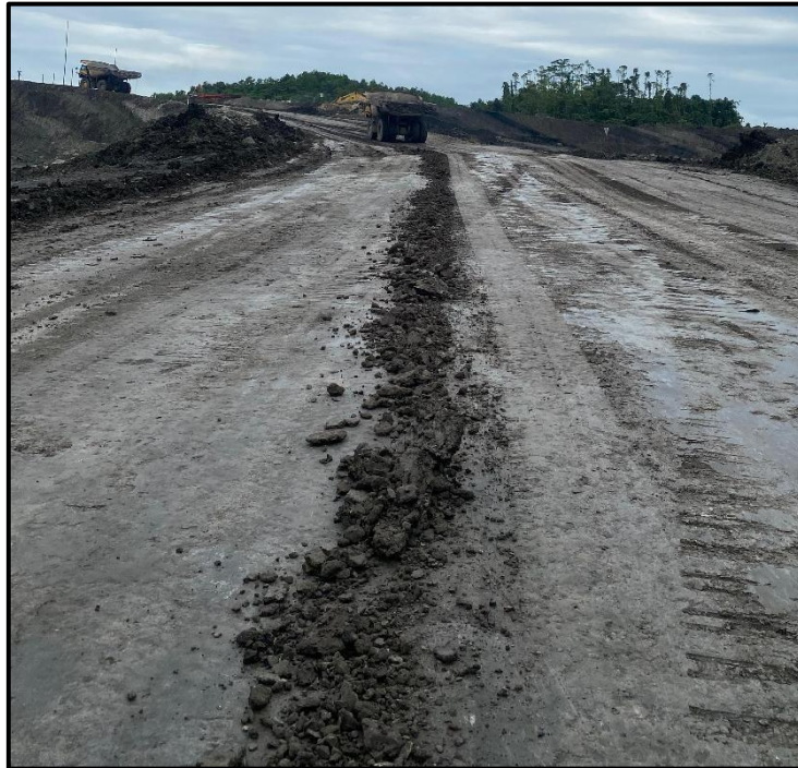
Gambar 9. Loose Aggregate
