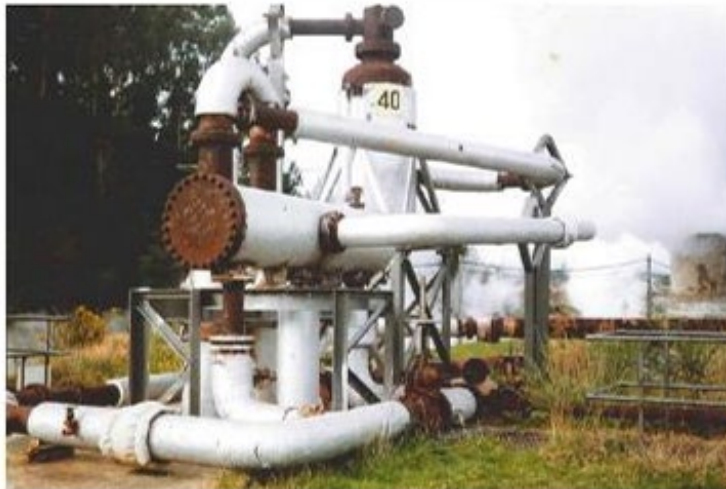
Gambar 3.1. Vertical Cyclone Separator
