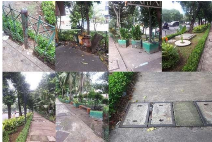
Figure 4. Existing condition of the study area (Documentation 2022)
