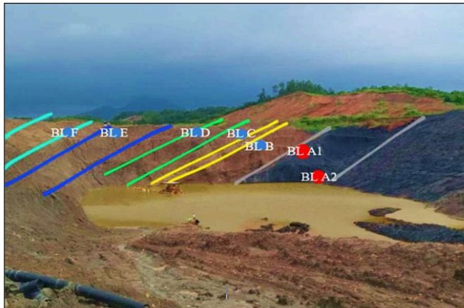
Figure 4. Distribution of PAF and NAF in the West Pit of PT Batubara Lahat
