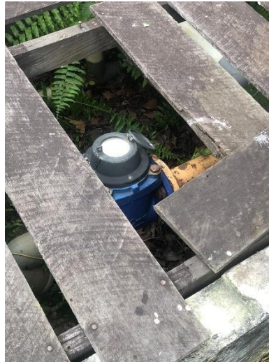
Gambar 4.20 Inspeksi Water Withdrawal Di area PMR
