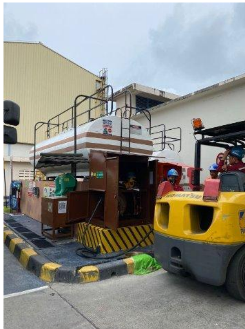
Gambar 4.29 Inspeksi GHG Reduction dan Renewable Energy
